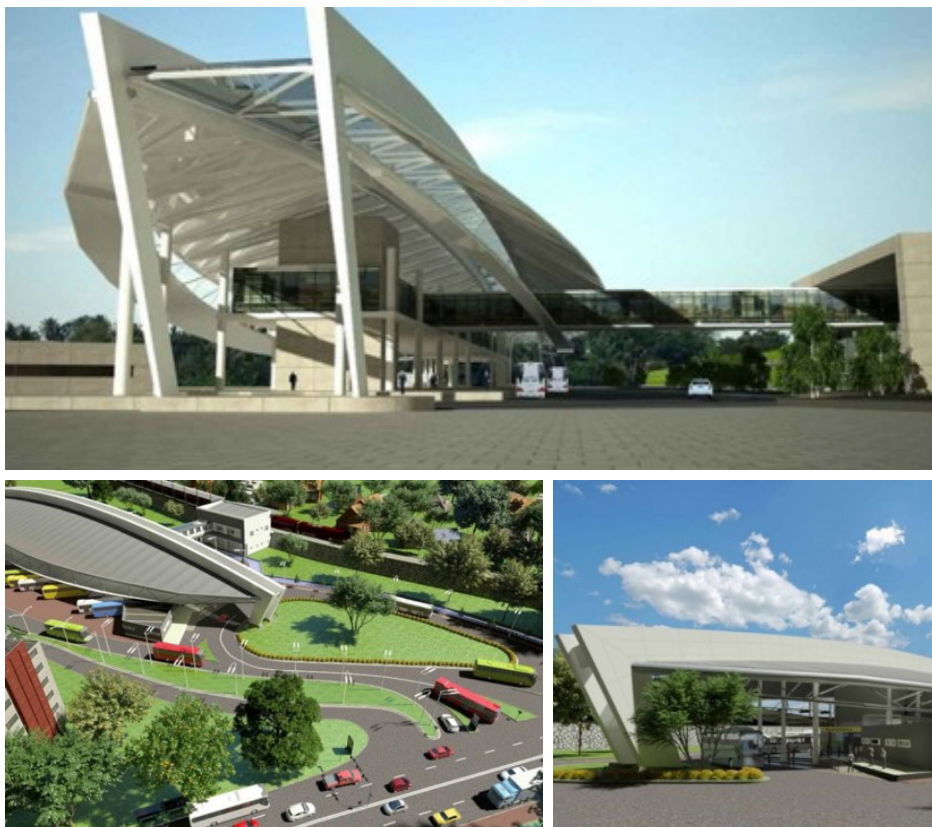
Figure 3.24 : Makubura Interchange Township Development Project Source : www.skyscrapercity.com
